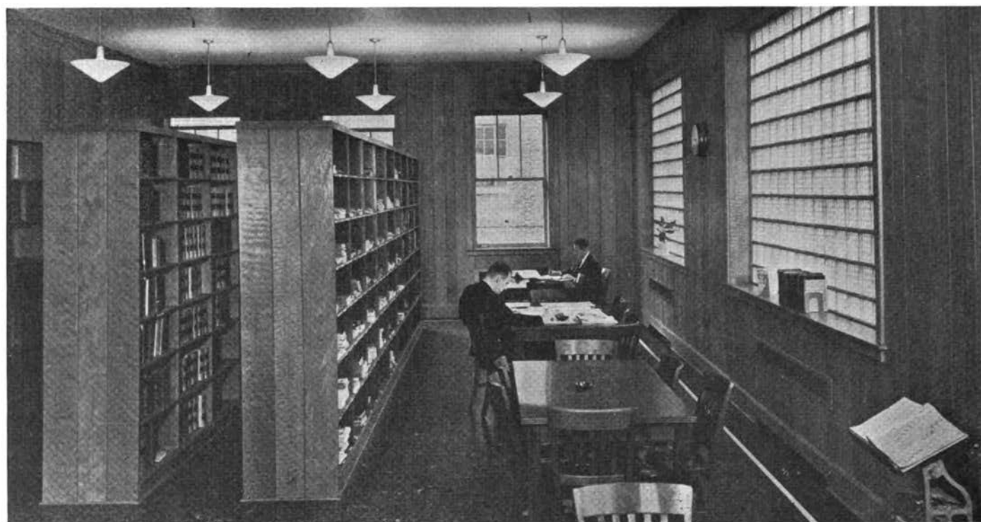
FIGURE 8.—Library, Research and Development Laboratories, Bakelite Corporation, Bloomfield, New Jersey. (Unit of Union Carbide and Carbon Corporation)
