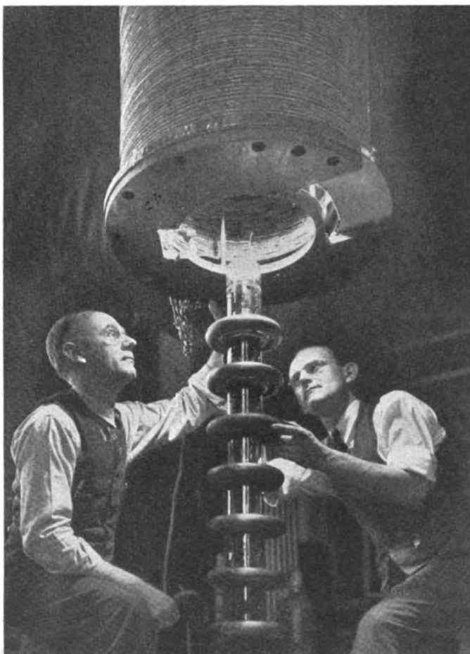
FIGURE 95.—Assembling of Million-Volt X-ray Unit, General Electric Company, Schenectady, New York
