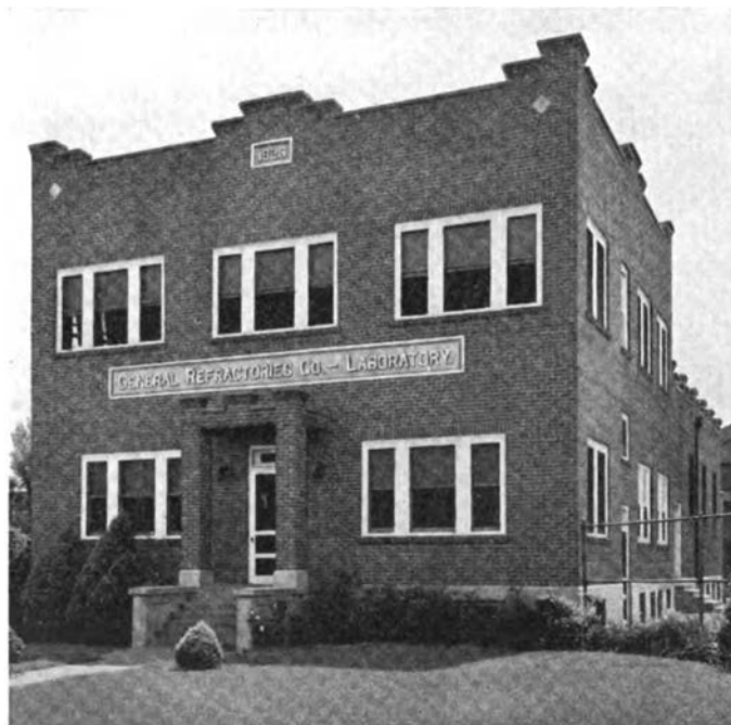
FIGURE 11.—Laboratory for Developing and Testing Refractories, General Refractories Company, Baltimore, Maryland
