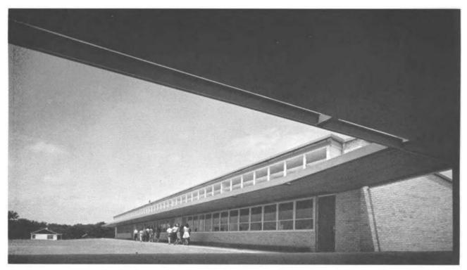
Fig. 4.3 I—Low glass area used for visual aid and light, protected by overhang; high glass area used for light only with interior horizontal sun control louvers, Westwood Elementary School, Stillwater, Okla.
