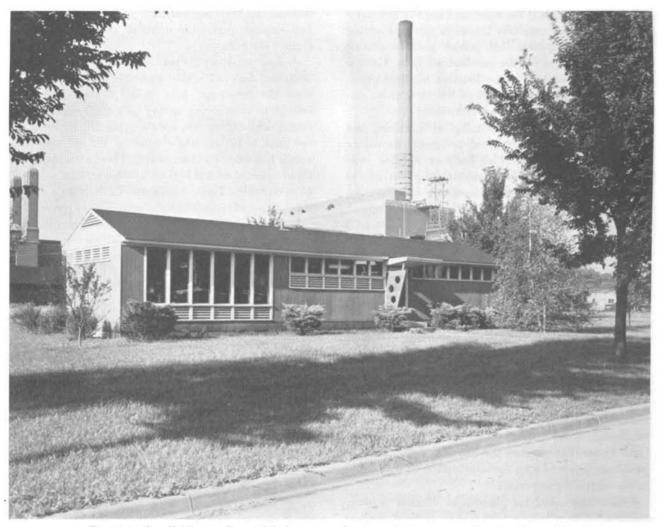
Fig. 4.4—Small Homes Council Laboratory showing windows on north elevation with ventilating units underneath fixed glass.
