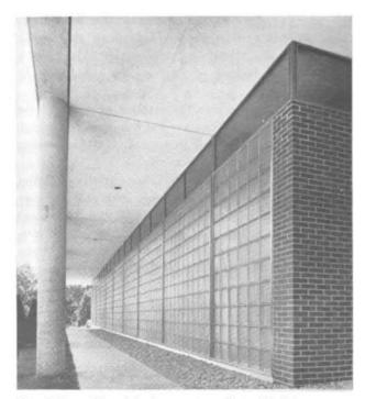
Fig. 2.21—Glass block curtain wall in Y.M.C.A., Port Chester, N. Y.
