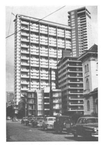
Fig. 1.24—Overhanging balconies, etc., on the southeastern exposure of an apartment house in Havana, Cuba.
