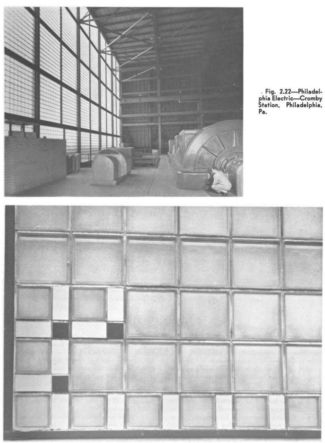
Fig. 2.24—Tile combined with two sizes of glass block for decorative effect.
