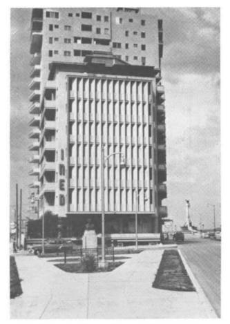
Fig. 1.27—Vertical concrete inclinded louvers on the western exposure of an apartment house in Havana, Cuba.
