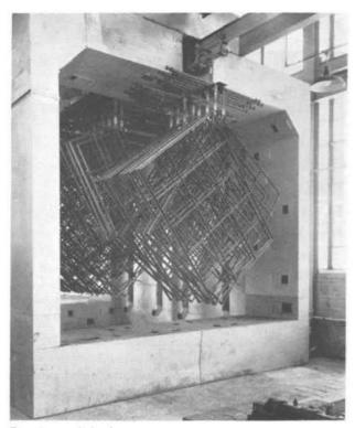
Fig. 2.15—Windows in drying oven after degreasing, pickling, rinsing and fluxing.
