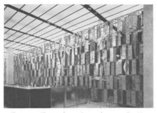
Fig. 3.5—This sculptured metal screen by Harry Bertoia acts as backdrop for the second floor. Of copper, brass and nickel fused to steel panels, it weighs six tons; is 70' wide, 16' high and 2' deep.
