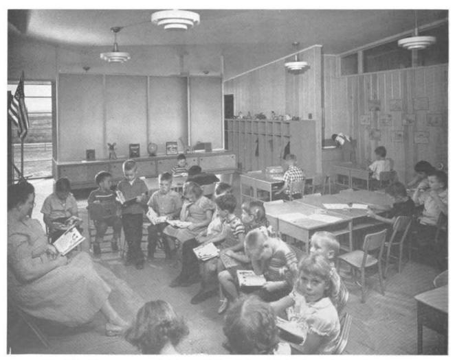
Fig. 4.28—Classroom separated from exterior window wall by glare-reducing glass screen.
