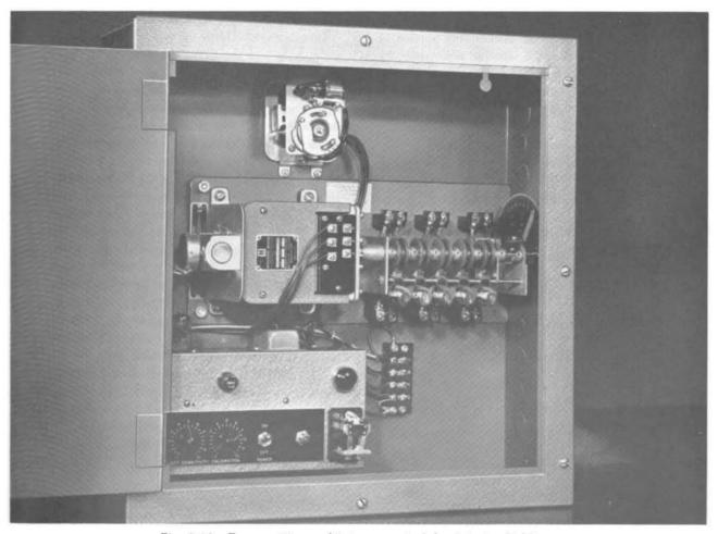
Fig. 3.18—Two position multi-stage control for interior lighting.
