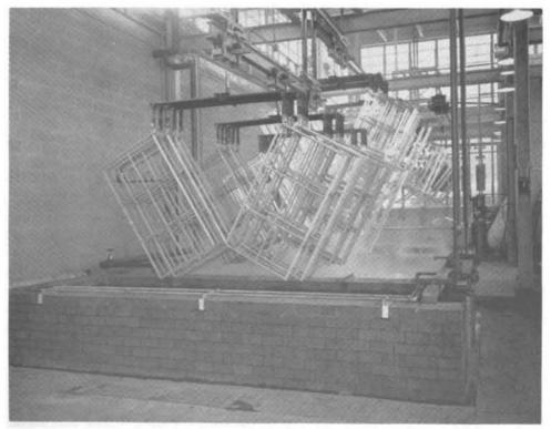
Fig. 2.17—Chemical treatment of windows after galvanizing.
