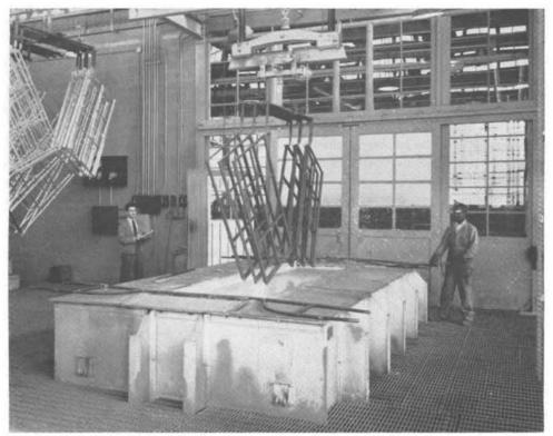
Fig. 2.16—Galvanizing bath, 110 tons of molten zinc.
