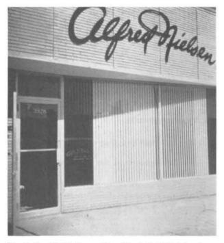
Fig. 3.14—Vertical venetian blinds installed in store front.
