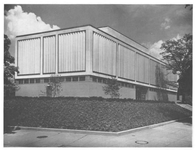
Fig. 1.28—Movable vertical louvers as used on the American Association for the Advancement of Science building in Washington, D. C.
