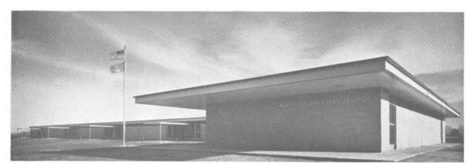
Fig. 4.30—Use of high brick walls on north and west with small glass area for light distribution, Madison Elementary School, Norman, Okla.
