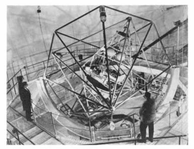
Figure 5. MASTIF simulator: a tumbling device on which astronauts experienced rotational rates up to 30 rpm in three axes. Once a steady rotational rate is achieved, astronaut assumes control and brings trainer to a stop by using instruments and controls similar to those available in Mercury vehicle.
