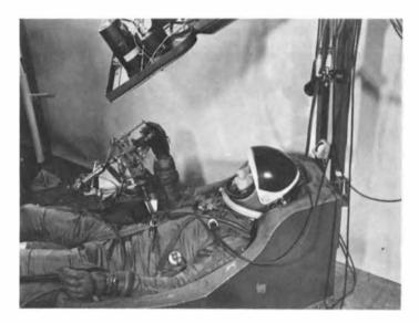
Figure 3. ALFA simulator: a dynamic simulator making use of an air bearing which provides practice in attitude control during orbit and retrofire phases of mission. External reference is simulated by use of a picture of earth from orbital altitude projected onto circular screen (seen behind trainer). Astronaut views screen through a set of mirrors and a lens which simulates periscope.
