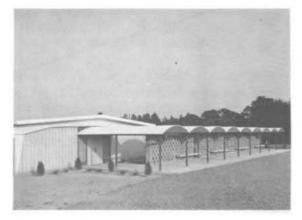
Fig. 10. Curved plywood panels form canopy
