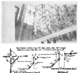
Fig. 11. Section of a completed electrical photo-drawing for a revision to an existing facility.
