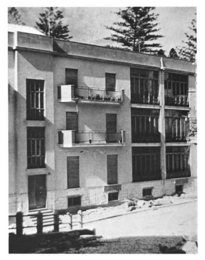
Figure 8. Santa Margherita di Belice. Modern apartment construction of a few stories height; reinforcedconcrete frame and slab, with masonry filler walls. Note cracks between frame and filler wall in first story.
