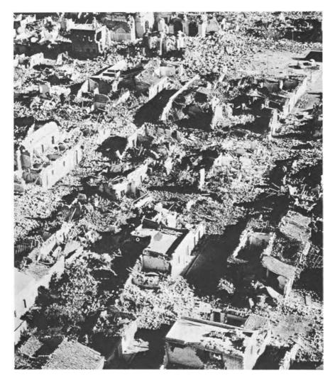
Figure 11. Montevago. At least two forms of construction are visible: an old rough masonry with polesupported tile roofs, and a newer cut-stone masonry with reinforced-concrete floors and roofs. The newer form seems to have fared somewhat better; nevertheless, the destruction in this view is almost complete. (Photograph courtesy of "Mondadori <u>Epoca</u>," Milan; photographers, "De Biasi - Del Grande - Lotti - Cioni.")
