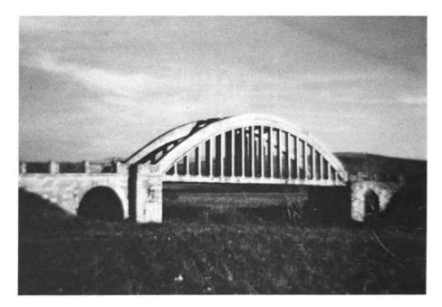
Figure 26. Highway bridge over the Belice River on road between Santa Margherita di Belice and Salaparuta. Reinforced-concrete tied-arch and suspenders; resting on cut-stone masonry abutment piers; span about 40 meters. The bridge suffered no apparent serious damage, and was in regular use by moderately heavy truck traffic. (View of west side of bridge).
