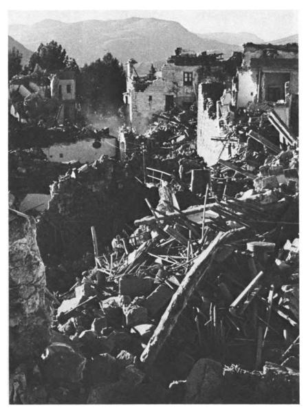
Figure 21. Collapsed houses, showing detail of some of the old forms of coarse masonry construction and building materials. (Photograph courtesy of "Mondadori <u>Epoca</u>," Milan; photographers, "De Biasi - Del Grande - Lotti - Cioni.")
