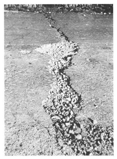
Figure 29. Crack across paved road surface on north fill approach near bridge shown in Figure 26. The vertical plane of the crack is approximately perpendicular to the longitudinal axis of the bridge.
