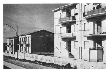
Figure 14. Outskirts of Montevago. Masonry and reinforcedconcrete slab construction. No apparent great damage.
