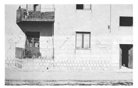
Figure 15. Outskirts of Montevago. Classic diagonal cracks in masonry walls. Considerable damage, although the building appeared to be repairable.
