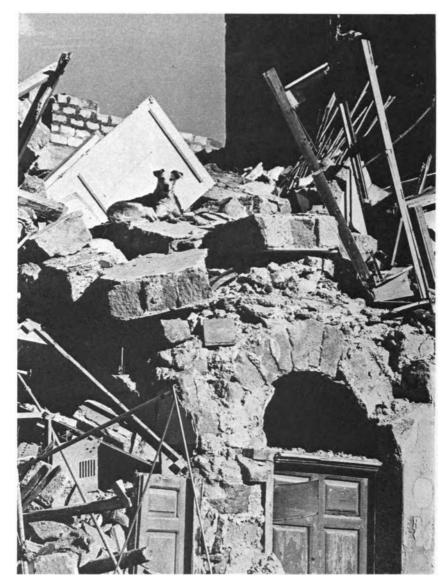
Figure 22. Collapsed building, showing the very heavy but weak masonry, heavily plastered and filled above the arch construction, the stones joined by very poor mortar. (Photograph courtesy of "Mondadori <u>Epoca</u>," Milan; photographers, "De Biasi - Del Grande - Lotti - Cioni.")
