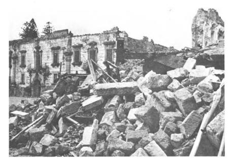
Figure 7. Santa Margherita di Belice. After the earthquake; the "Leopard's Palace" and adjoining church (compare Figure 6). The clock and parapet wall on the palace have fallen, but the facade still stands. The church is in complete ruins. (Source: "Scafidi" photographic agency, Palermo.)
