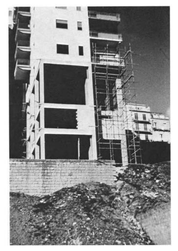
Figure 5. Salemi. Part of multistory, reinforced-concrete frame apartment building nearing completion. There were no outward signs of significant damage visible from the distance at which the picture was taken.
