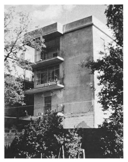
Figure 9. Santa Margherita di Belice. Rear view of a wing of the building shown in Figure 8. Note cracks between frame and filler wall and around lintel; fallen external plaster. The building apparently is repairable.
