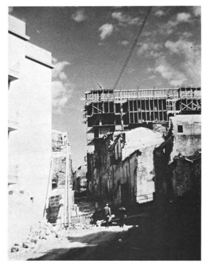
Figure 10. Santa Margherita di Belice. Corner of building at left is a portion of building shown in Figures 8 and 9. Building under construction in the distance is an eightstory, reinforced-concrete frame and slab structure with hollow tile filler walls. It showed (from a distance) no signs of serious damage. The other buildings in the picture were generally of old rough masonry construction and were very seriously damaged.
