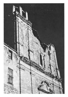
Figure 3. Vita. Church facade, showing fallen roof, wall and masonry ornamentation.
