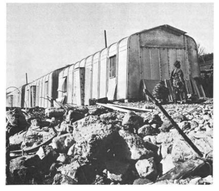
Figure 36. Temporary metal prefabricated housing being erected for family groups. (Source of photograph: "Scafidi" photographic agency, Palermo.)
