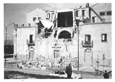
Figure 16. Near Montevago. Church-convent at Convento Madre di Grázie. Old rough-masonry facade backed by more recent construction consisting of reinforced-concrete frame and masonry. The fallen concrete beams and slab evidently were supported by the old masonry construction at the front. The reinforced-concrete frame structure at the rear appeared to be repairable.
