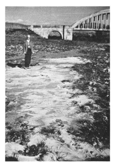
Figure 30. Sandboil area on the north bank of the Belice River, west of the bridge shown in Figure 26. The line of the sandboils is approximately east-west.
