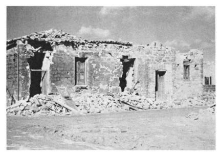
Figure 12. Montevago. Older type of construction; rough masonry with pole-supported tile roofs.
