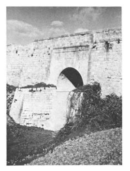
Figure 24. Near Salemi. Old highway bridge. No outward signs of great damage, but we were told that the bridge was to be removed and replaced by a culvert and fill.
