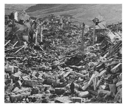
Figure 19. Gibellina. Complete destruction. The construction appears to have been somewhat more substantial than that in Salaparuta, but no less subject to damage. (Photograph courtesy of "Mondadori <u>Epoca</u>," Milan; photographers, "De Biasi - Del Grande - Lotti - Cioni.")
