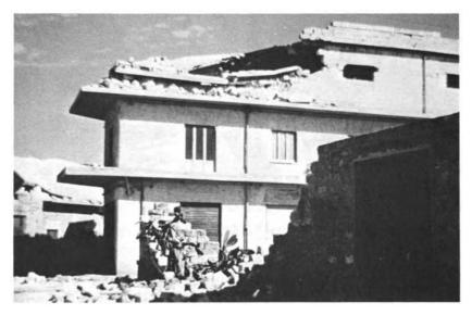
Figure 13. Montevago. Newer construction with cut-stone masonry, concrete lintels, and reinforced-concrete floor slabs.
