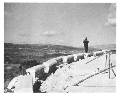
Figure 28. Road between Salemi and Montevago. Masonry guard walls on filled road shoulder shifted or overturned; cracks in road surface.
