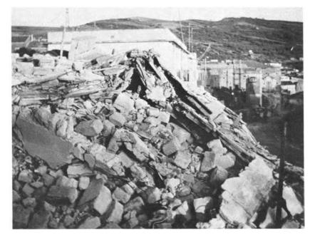
Figure 17. Poggioreale. Complete collapse of a building alongside another, still standing, of apparently similar age and construction. The collapsed building apparently contained a very poor grade of reinforced concrete. Note the collapsed floor slabs of reinforced concrete and hollow tile.
