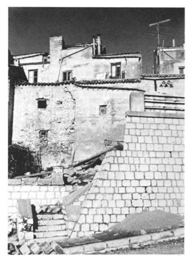
Figure 4. Vita. Showing old and new construction of local stone. The new wall in the foreground appeared to have been well constructed. The old walls are of very coarse, crude masonry with ineffective mortar.
