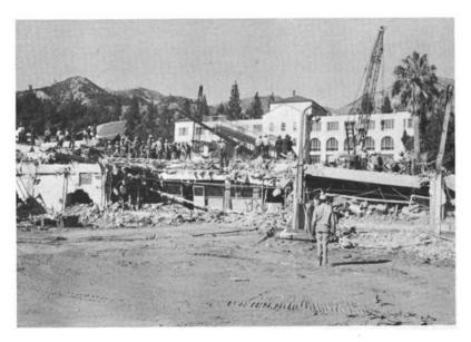
FIGURE 4 Collapsed portion of Sylmar Veterans Hospital being removed in search for survivors. The last of 14 survivors was found shortly after this photograph was taken. In this Hospital, built before the current building codes were established, 42 people were killed. Photograph courtesy of Earthquake Engineering Research Laboratory, California Institute of Technology.
