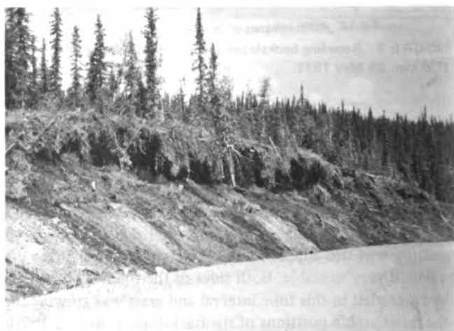
FIGURE 12 Slope has receded to edge of clearing in Figure 11, 32.6 km, 11 August 1970.
