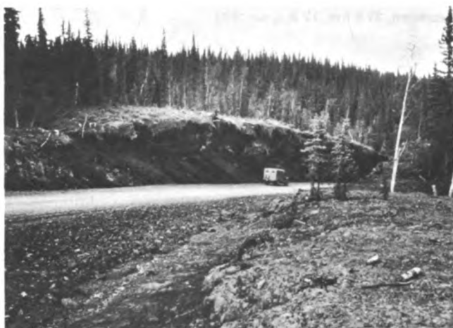
FIGURE 11 Overhanging mat and clearing atop backslope, 32.6 km, 26 June 1970.
