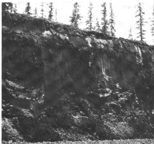
FIGURE 9 Frozen vertical backslope, 32.6 km, 23 April 1970.
