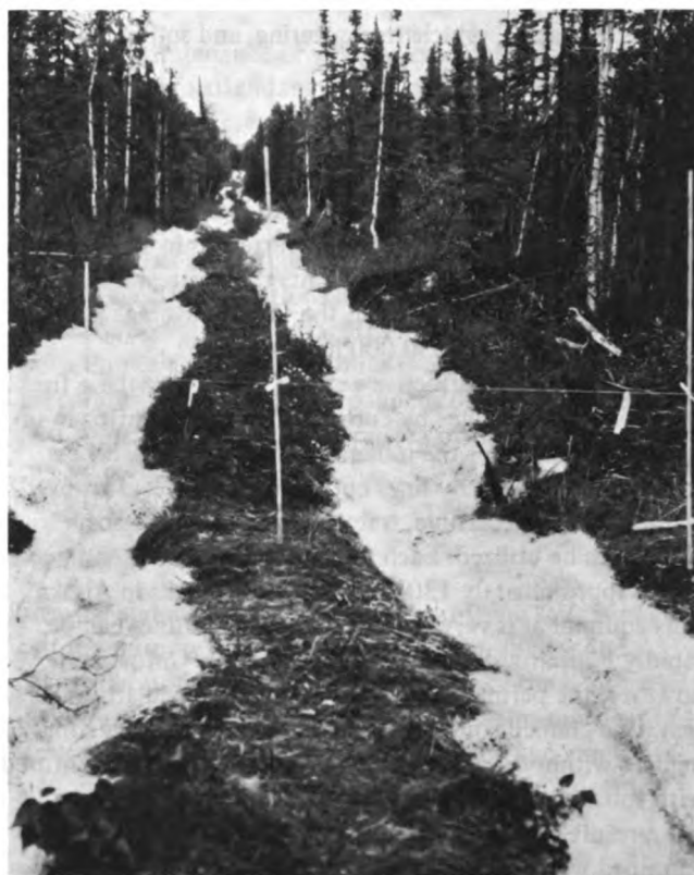
FIGURE 4 Same trail identified in Figure 3 after application of seed and fertilizer covered by excelsior mulch.
