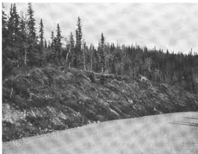
FIGURE 16 More stable backslope, 32.6 km, 17 August 1971.
