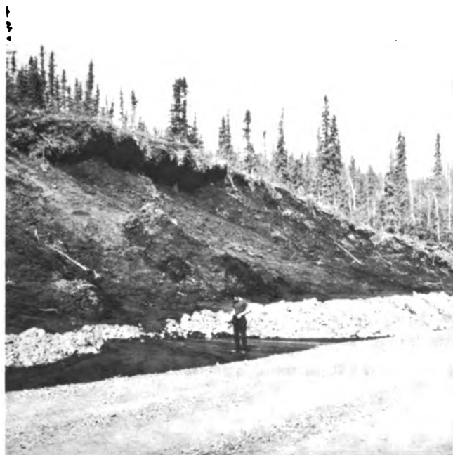
FIGURE 7 Receding backslopes and stabilized ditch sediments, 31.6 km, 28 May 1971.
