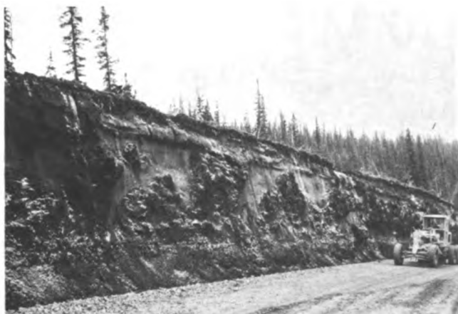
FIGURE 10 Frozen vertical backslope, 32.6 km, 23 April 1970.
