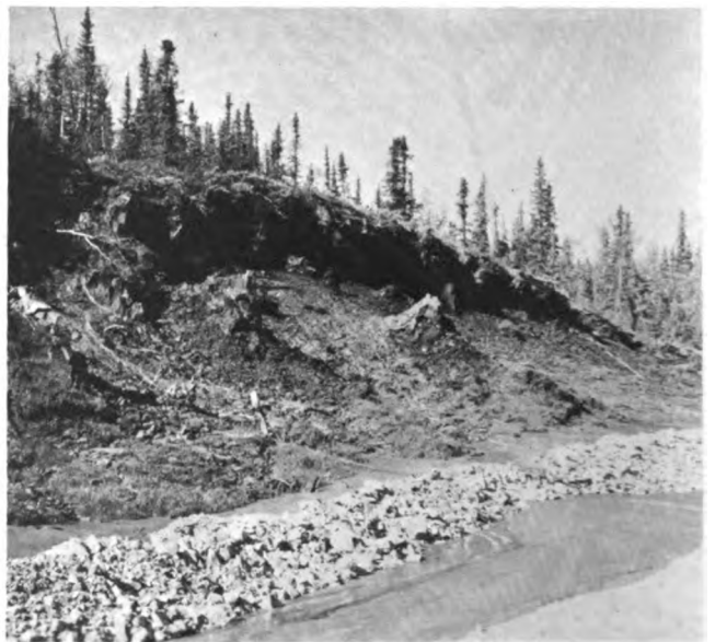
FIGURE 6 Seeded backslope and broken rock revetment, 31.6 km, 11 August 1970.
