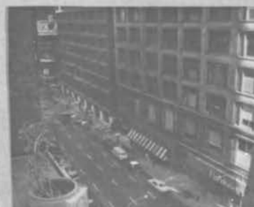
BLOCK 8 (elevated view) NORTH
