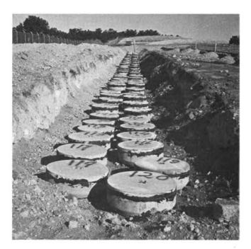
FIGURE 18 Concrete casks for storing drums of waste contaminated with plutonium-238 are sealed before being covered with 2 meters (6.6 feet) of crushed tuff and soil in Area G at the Los Alamos Scientific Laboratory.
