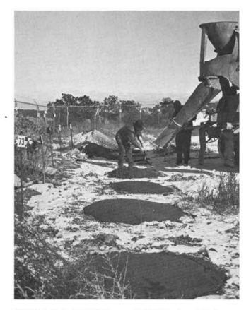
FIGURE 4 Shafts,  $0.75 \times 0.75$  meters ( $2.5 \times 2.5$  feet), are drilled into the tuff in Area G at the Los Alamos Scientific Laboratory to dispose of solid waste that requires shielding. Some of the shafts are concrete lined. A sealing plug of concrete 1 meter (3.3 feet) thick is poured when the shaft is full.
