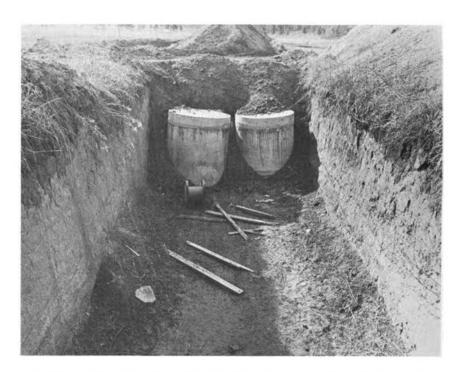
FIGURE 14 Transuranium-contaminated waste in steel drums was originally sealed in concrete casks  $2 \times 2$  meters (6.6  $\times$  6.6 feet) and retrievably stored in trenches up to 6 meters (20 feet) deep at the Savannah River Plant.
