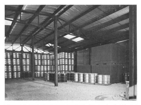
FIGURE 10 Transuranium waste with low external gamma radiation is packaged in stainless steel drums and stored in a corrugated metal building at the Oak Ridge National Laboratory. A reinforced concrete and concrete block pit-type structure is under construction; this waste will be transferred to the new structure when it is completed.
