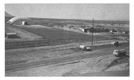
FIGURE 8 On the left is shown an air support structure erected over the first cell of the second pad in the Transuranic Storage Area (TSA) at the Idaho National Engineering Laboratory. To the right is shown the final cell of the first pad being completed. Note that an airlock permits truck access to the air support structure without disturbing operations.
