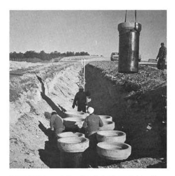
FIGURE 16 Waterproofed concrete cylinders are placed into trenches  $(122 \times 9.2 \times 6.1 \text{ meters}, \text{ or } 400 \times 30 \times 20 \text{ feet})$  in Area G at the Los Alamos Scientific Laboratory to retrievably store waste contaminated with plutonium-238. Topsoil is about 0.6 meters (2 feet) thick over tuff. The water table is 275 meters (900 feet) below the surface.
