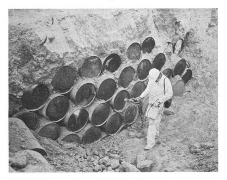
FIGURE 20 A health physicist monitors 210-liter (55-gallon) drums of transuranium-contaminated waste for external contamination before they are removed as part of a study program after being buried for 5 years at the Idaho National Engineering Laboratory. Almost all of the drums are intact.
