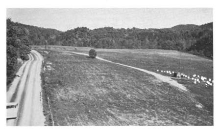
FIGURE 3 The Solid Waste Storage Area 4 at the Oak Ridge National Laboratory after it was no longer in use for burials. The burial area has been contoured and planted with grass. It occupies about 9.3 hectares (23 acres).
