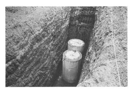
FIGURE 11 Transuranium-contaminated waste at the Oak Ridge National Laboratory that has high gamma radiation levels is sealed in reinforced concrete casks 1.4 meters (4.6 feet) in diameter and 2.4 meters (7.9 feet) long having wall thicknesses from 12 to 30 centimeters (4.7 to 12 inches), depending on the shielding required. Casks are retrievably stored below grade in trenches 3 meters (10 feet) deep.
