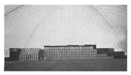
FIGURE 9 An air support structure over the first cell on the second pad of the Transuranic Storage Area at the Idaho National Engineering Laboratory protects the waste from the weather and allows year-round operation. When the cell is complete, the air support structure will be moved to cover the second cell, and the first cell will be covered with plywood, a waterproof membrane, and 1 meter (3 feet) of soil.
