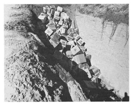
FIGURE 2 Solid waste with very low levels of radioactivity (near background level) is disposed of in cardboard boxes into trenches 6 meters (20 feet) wide and 6 meters (20 feet) deep at the Savannah River Plant. Trenches are backfilled periodically, then finally covered with 1.2 meters (4 feet) of soil when full. The soil is a mixture of sand and clay; the distance to the water table is 13 meters (43 feet).
