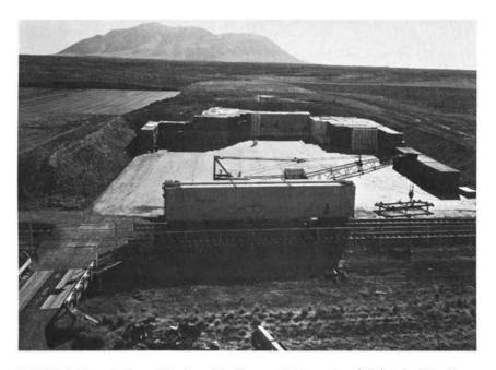
FIGURE 6 Shown is the working face of the Transuranic Storage Area (TSA) at the Idaho National Engineering Laboratory. Waste arrives by truck or in special railcars and is stacked on an asphalt pad  $45 \times 730$  meters ( $150 \times 2,400$  feet) in cells 24 meters (80 feet) deep. When a cell is complete, the cell is covered with plywood, a waterproof membrane, and soil, and is then seeded to prevent wind erosion. Initial construction of a second pad is shown on the left.
