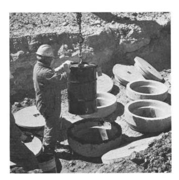
FIGURE 17 Drums (115 liters or 30 gallons) of waste containing more than 100 nanocuries of plutonium-238 per gram of waste are placed into waterproof concrete casks for retrievable storage in Area G, at the Los Alamos Scientific Laboratory. Each cask contains two drums.
