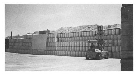
FIGURE 7 Drums (210 liters or 55 gallons) of transuranium-contaminated waste are stacked on an asphalt pad at the Idaho National Engineering Laboratory in the Transuranic Storage Area (TSA) for retrievable storage. The drums and coated boxes are covered with flame-resistant plywood and reinforced plastic sheets before being covered by 1 meter (3 feet) of soil for protection from the weather.
