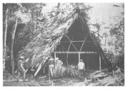
FIGURE 8 Low-Technology Shelter Solutions: An example of low-technology solutions is the Intertect/Carnegie-Mellon University A-frame emergency housing shown here being field tested in Guatemala. The system was subsequently used in Bangladesh refugee camps.
