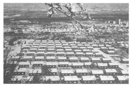
FIGURE 10 Prefabricated Housing: These prefabricated housing units in Skopje, Yugoslavia, were built within 8 months following the earthquake of 1963.
