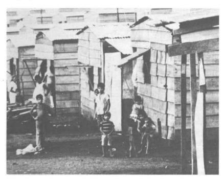
FIGURE 9 Low-Technology Solutions: A total of 11,000 of these U.S. AID wooden housing units were built in Managua, Nicaragua, within 3 months of the disaster there. They were described as temporary when built, but they have inevitably become permanent.
