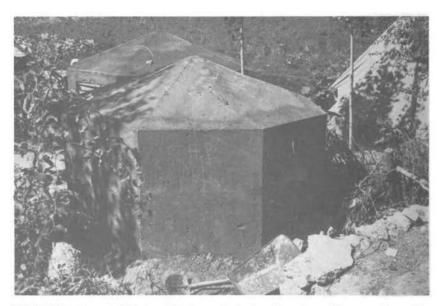
FIGURE 12 Imported Shelter Solutions: Oxfam's polyurethane igloos are pictured in use in Lice, Turkey, following the 1974 earthquake. By the time these "temporary" units arrived, 60 days after the disaster, the 1,500 "permanent" prefabricated houses had been completed (see Figure 11).
