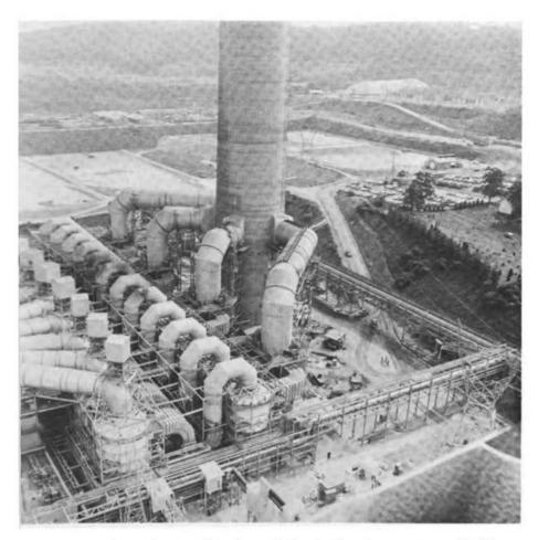
ubber system for units 1 and 2 at the Bruce Mansfield i to remove 99.8 percent of the fly ash and 92.1 percent xide. The scrubbers require 5 percent of each unit's cost approximately \$13 million a year per unit to ;ain. (Photo courtesy Pennsylvania Power Company.)
