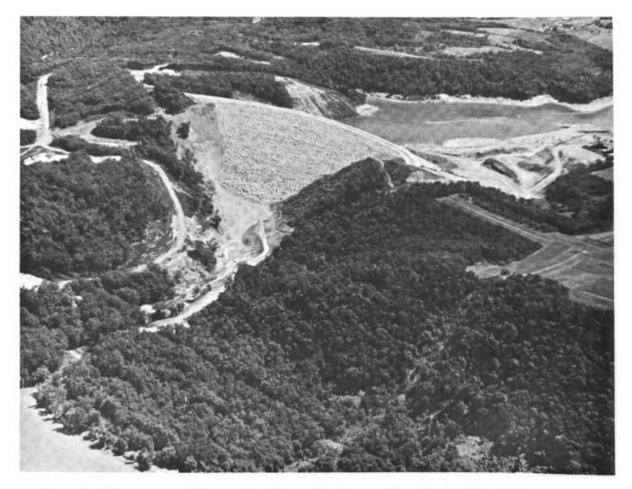
FIGURE 4 The gypsumlike waste from the Bruce Mansfield Plant is deposited in the valley behind the dam. The capital cost of this wastedisposal system is reported to be \$90 million. (Photo courtesy Pennsylvania Power Company.)
