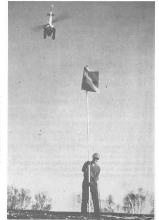
Gogama District, Ontario. Helicopters require a power-driven centrifugal slinger for distributing the seed. The types in use in North America cover a swath 30 m wide. Flagmen are often used to guide helicopters and ensure that seed is spread evenly. (J. Scott)
