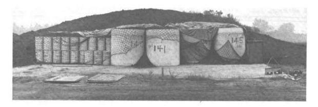
FIGURE 5 Storage pad and container for TRU alpha waste.
