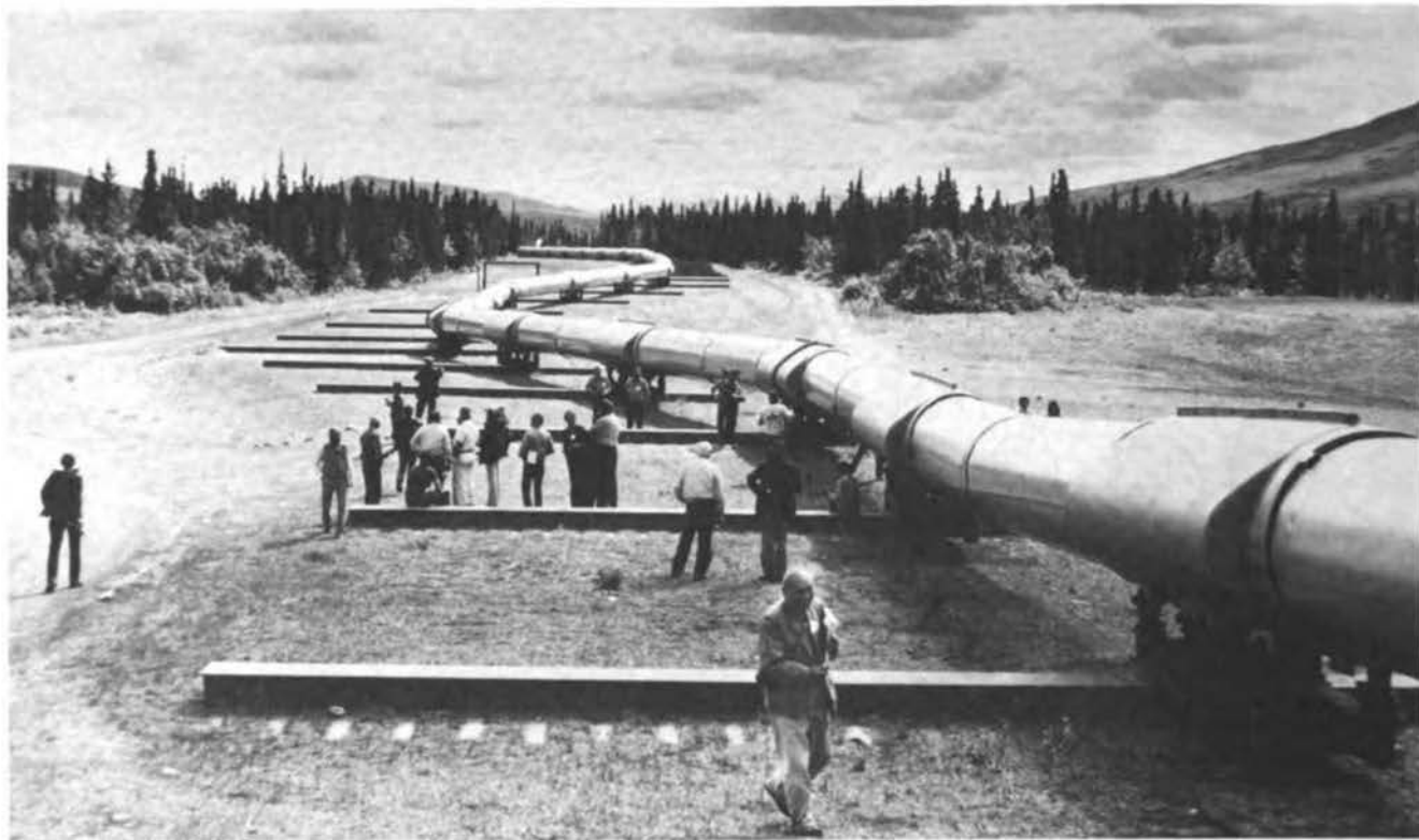
Participants of B-4 field trip at the trans-Alaska pipeline crossing the active Denali fault, central Alaska Range, one of the largest crustal breaks in Alaska. Average rate of displacement along the Denali fault is 0.1 to 3.5 cm per year; 5 to 60 m of right-lateral movement and 6 to 10 m of vertical movement have occurred during the past 10,000 years. The pipeline is so constructed here that it can slide laterally as much as 6 m on Teflon "shoes" to accommodate lateral displacement along this right-lateral, strike-slip fault. It can also accommodate 1.8 m vertical displacement. The 1.2-m-diameter warm-oil pipeline was completed in 1977 and no serious maintenance problems have developed along the 1,285-km route over permafrost terrain. (Photograph No. PK25557 by T.L. P  w  , July 24, 1983.)
