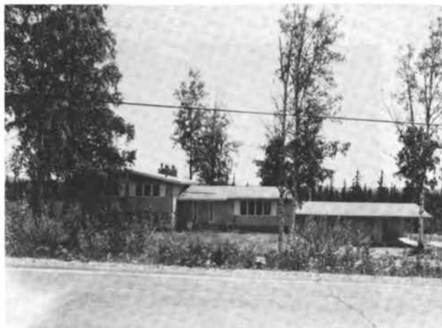
Stop 4. House built in 1975 on ice-rich permafrost. (Photograph 3997 by T.L. Péwé, 1977.)
