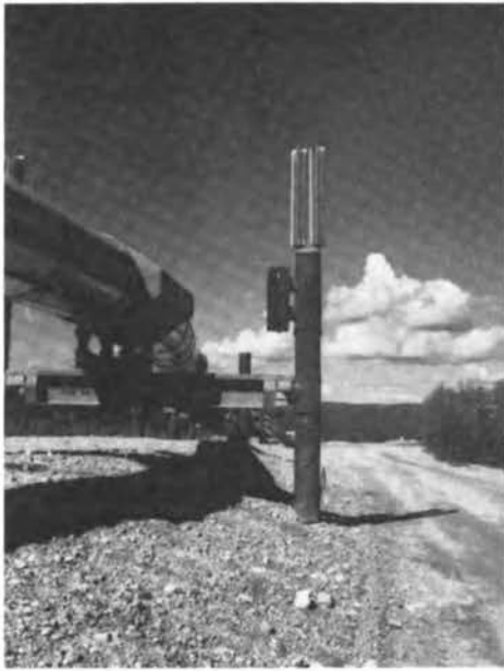
Stop 5. Elevated section of Trans-Alaska Pipeline at Engineer Creek, 5 miles north of Fairbanks. The pipe is insulated with 4 inches of resin-impregnated fiberglass jacketed by galvanized steel. (Photograph 3986 by T.L. Péwé, July 17, 1977.)
