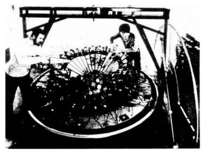
Figure 4.2 One hemisphere of the Plastic Ball detector during its assembly. Consisting of 815 pyramidal scintillator detector modules, each with its own electronics package, the complete detector covers 96 percent of the total solid angle into which nuclear-reaction products can be emitted. (Courtesy of the GSI/LBL Collaboration, Lawrence Berkeley Laboratory.)
