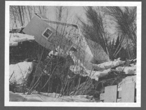
Earthquakes often trigger massive landslides, such as the one shown here in the Turnagain Heights subdivision in Anchorage, Alaska. The great Alaskan earthquake of March 1964 (magnitude 8.4), liquified sand lenses beneath the subdivision, causing a complex slide with severe surface contortion. During the four minutes of perceptible ground shaking, the front of the slide moved more than 1,000 ft, destroying 35 homes. (Source: G. W. Housner, California Institute of Technology.)
