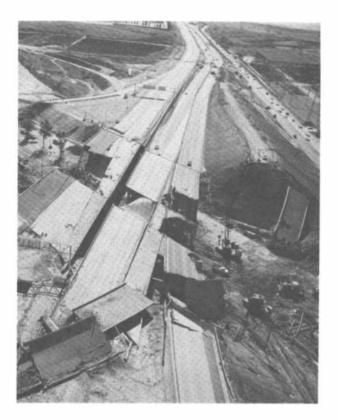
On February 9, 1971, the magnitude 6.5 San Fernando, California, earthquake damaged 42 freeway bridges and collapsed five, including these in the Sylmar region of Los Angeles. Since then, California highway officials have required overpass designs to incorporate dynamic analyses and the results of extensive earthquake engineering research. (Source: G. W. Housner, California Institute of Technology.)
