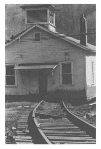
Transported by flood waters from its original site along Buffalo Creek, this local church ended its journey straddling damaged railroad tracks. In addition to the loss of life and personal property it caused, the Buffalo Creek flood also destroyed critical infrastructure elements, such as power, water, and sewer facilities, bridges, highways, and rail lines. (Source: Uniphoto.)
