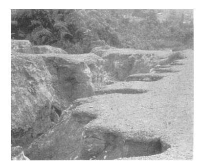
Roads commonly spawn severe erosion. The smooth, flat surface collects water and cascades it over the banks, washing out the slopes below. Slopes above the road are also erosion prone, especially as they are often extremely steep. Embankments freshly cut out of hillsides or built up from fill are particularly vulnerable. The damage can be immense—to the roads, to the neighbors, and to the environment in general.
