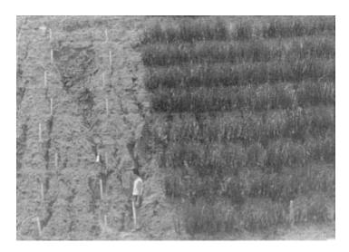
Rows of vetiver were able to stabilize fill dirt within a few weeks of planting. Although not really established in the loose and highly erodible soil, they protected the site during one of the severest downpours in memory. The bare section adjacent washed out. (P.K. Yoon)
