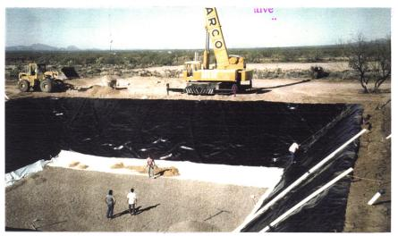
This photograph shows a lined basin constructed at the University of Arizona's Avra Valley Geophysical Test Site. The basin is 30 m by 30 m by 5 m deep. The entire basin was lined with high-density polyethelene; drain pipes were placed in the bottom and the basin refilled with native soil. This test site allows a closed system for injection and retrieval of fluids. During the summer of 1992, 24,170 liters of water were injected along a 1-m by 25-m strip at the center of the basin.
