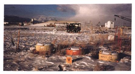
Photograph shows a survey being conducted at a site at a radioactive waste management acid pit at the Idaho National Engineering Laboratory. The site had been used for dumping acid that contained radioactive wastes and other contaminants. This was an operational survey to provide information for remediation of the site, and the precise location of the wastes were not well known.
