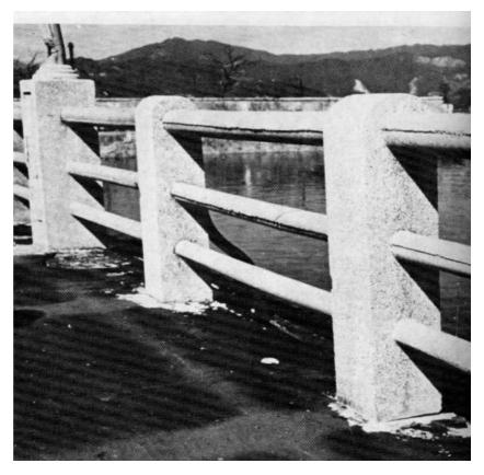
FIGURE 2-2 Flash marks produced by thermal radiation on asphalt of bridge in Hiroshima. Where the railings served as protection from the radiation, there were no marks; the length and direction of "shadows" indicate the point of the bomb explosion (Glasstone and Dolan 1977).
