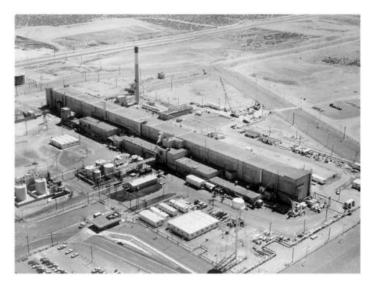
FIGURE 2.4 Chemical separation of plutonium from other radioactive materials was carried out in Hanford's PUREX plant and similar facilities. They were referred to as canyons because thick walls to protect workers from radiation surrounded the long, remotely operated processing corridor. Source: http://www.fas.org/irp/imint/doe.htm
