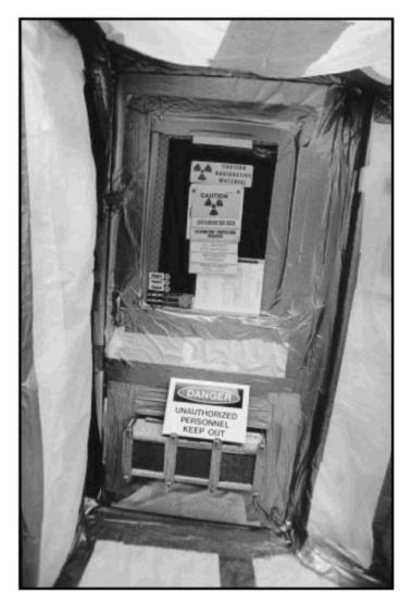
FIGURE 2.6 Door leading into a plutonium processing room at the Rocky Flats Site is sealed due to very high levels of alpha radiation within the room. There are more than 20 such rooms at the site. Source: DOE, 1996.
