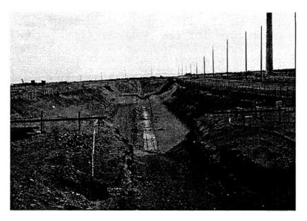
Figure 2.5 Construction of a drainage crib at the Hanford Site in 1944. The sawhorse in the excavation provides scale. SOURCE: David Briggs, Pacific Northwest National Laboratory, Negative 3543.
