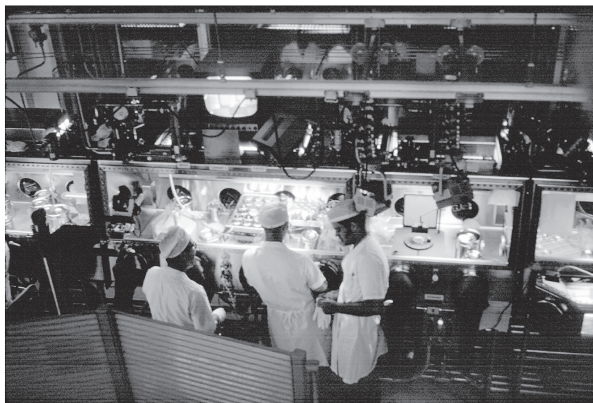
FIGURE B.2 A portion of the sterile nitrogen atmospheric processing (SNAP) line, a system of glove boxes used for processing samples returned by the later Apollo missions. The cabinets contain purified dry N 2 at slightly more than atmospheric pressure, so leakage is outward, protecting the samples but not personnel (if the samples had contained pathogens). Gas in the cabinets is continuously monitored for contamination by organic compounds, water vapor, oxygen, and other trace gases. SOURCE: Photograph by J.A. Wood.
