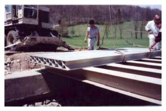
FIGURE 48 Placement of FRP deck modules over FRP stringers (Laurel Lick Bridge). [Source: Shekar et al. (34).]
