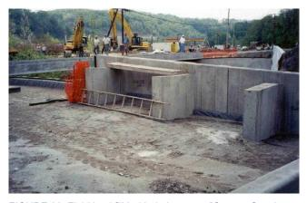
FIGURE 36 Fluid backfill behind abutment. [Source: Scanlon et al. (26).]
