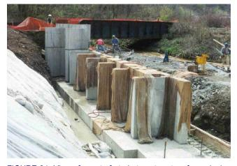
FIGURE 34 View of counterfort abutment system for a singlespan bridge over Miller's Run Creek in southwestern Pennsylvania. [*Source*: Scanlon et al. (26).]
