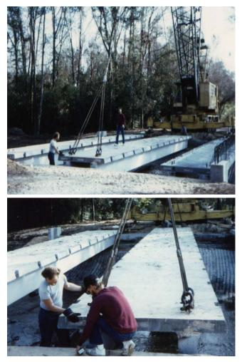
FIGURE 33 Construction of transversely posttensioned double-tees bridges.
