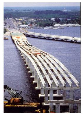
FIGURE 40 View of prefabricated substructure and girders of Edison Bridge.
