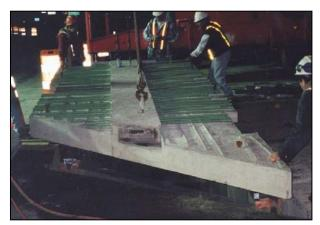
FIGURE 29 Installation of new panel of bridges at Route 7 over Route 50, Fairfax, Virginia. [Source: Babaei et al. (1).]
