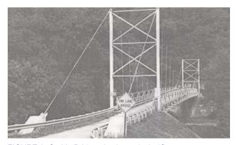
FIGURE 3 Corbin Bridge aluminum deck. (*Source:* www. aluminum.org/Content/NavigationMenu/The\_Industry/Building\_ Construction\_Market/Bridges/Bridges.htm.)
