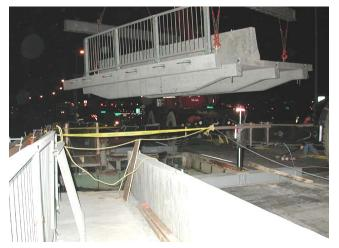
FIGURE 43 Prefabricated deck panel. (Source: www.pjcci.ca.)
