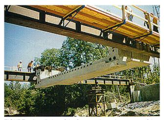
FIGURE 4 Installation of the first two channel segments of the Carpenter Road Bridge. (*Source*: http://www.tfhrc.gov/pubrds/ septoct98/channel.htm.)
