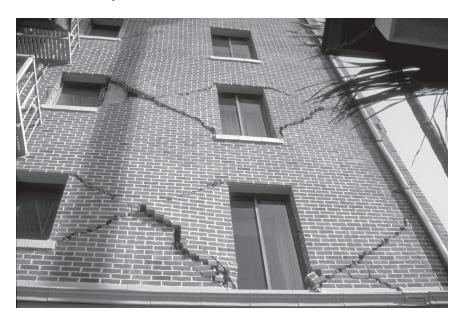
FIGURE 2.6 Structural damage to masonry building resulting from the 1994 Northridge, California, earthquake. Reproduced courtesy of the National Information Service for Earthquake Engineering, University of California, Berkeley.
