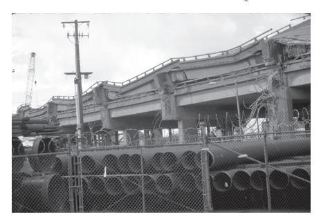
FIGURE 2.5 Collapse of the Cypress Avenue Freeway, 1989 Loma Prieta, California, earthquake. Reproduced courtesy of the National Information Service for Earthquake Engineering, University of California, Berkeley.
