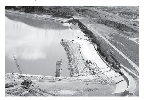
FIGURE 2.4 Embankment failure due to liquefaction at the Lower Van Norman Dam, 1971 San Fernando, California, earthquake. Reproduced courtesy of the National Information Service for Earthquake Engineering, University of California, Berkeley.
