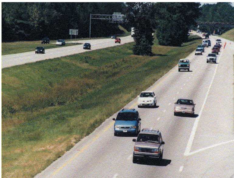
FIGURE 3-22 Contraflow along I-26 near Charleston, South Carolina, during reentry after Hurricane Floyd in September 1999. SOURCE: South Carolina Department of Transportation.
