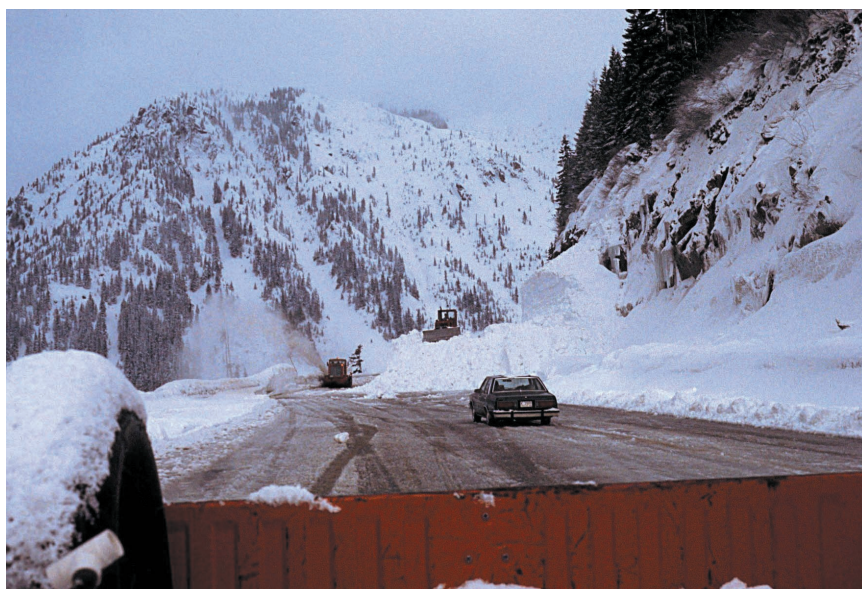
FIGURE 4-4 Removal of avalanche debris along US-2 in Washington. SOURCE: Northwest Weather and Avalanche Center, Seattle, Washington.
