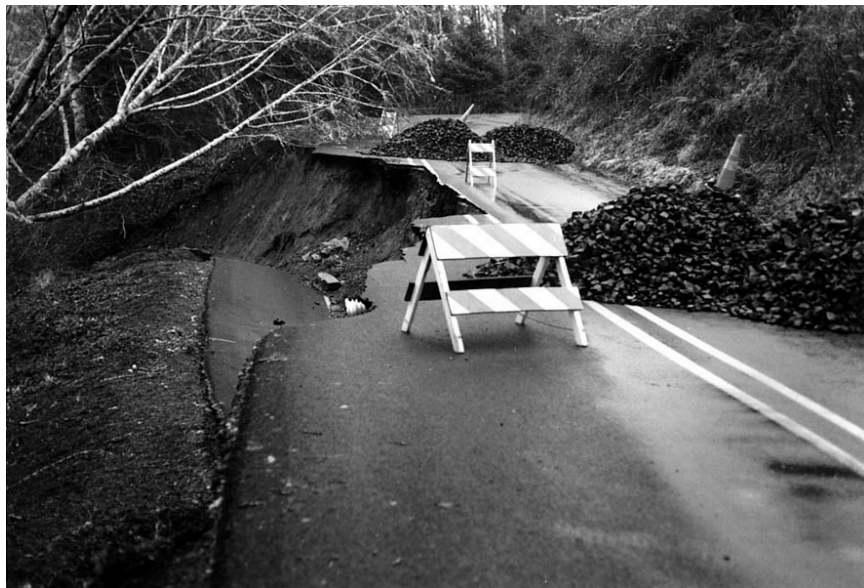
FIGURE A.4 Damage from the head scarp of a small earth slide closed Oregon State Highway 229, 13 miles north of Siletz, Lincoln County, Oregon. The landslide is typical of the numerous landslides caused by heavy winter rains in November and December 1998 in the Pacific Northwest. SOURCE: Baum and Chleborad (1999).
