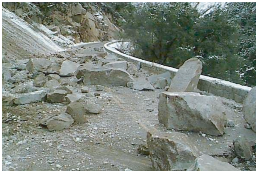
FIGURE A.5 Rock fall damage to El Portal Road, Yosemite National Park, February 12, 2001.
