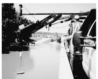
Figure 32. Sounding weight with wireless sonar.
