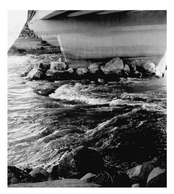
*Figure 42. Flow conditions between the right abutment and Pier 2.*
