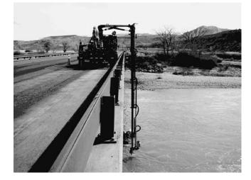
*Figure B1.* Crane on downstream side of bridge near scour hole.
