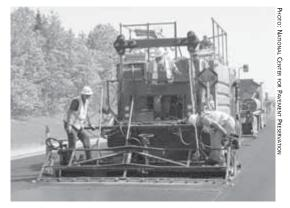
Microsurfacing is one of many pavement preservation techniques that states are integrating into a plan of preventive maintenance, rehabilitation, and reconstruction.
