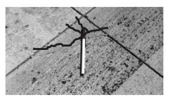
FIGURE B15 Typical UTW deflection spalling at the FHWA ALF.
