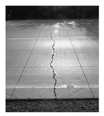
FIGURE 32 Typical midpanel crack on a TWT.
