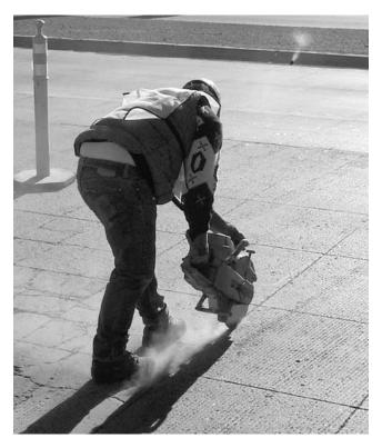
FIGURE 38 UTW repair step 1-Outline sawing.
