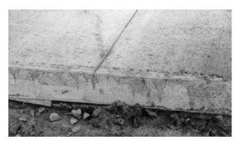
FIGURE 25 Sawcut depth using an early-age saw.
