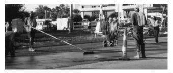
FIGURE 20 Application of texture with a coarse broom.
