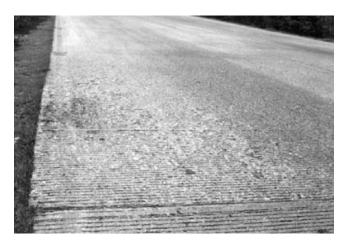
FIGURE 37 Typical surface wear.
