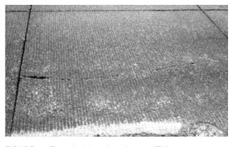
FIGURE 33 Typical midpanel crack on a UTW.
