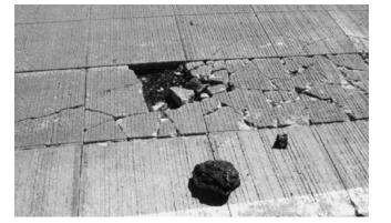
FIGURE 35 Severely shattered slabs on a UTW.
