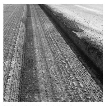
FIGURE 7 Milled HMA surface before overlay.
