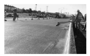
FIGURE 18 Water sheen on a concrete surface.
