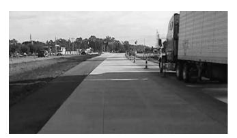
FIGURE 27 New shoulders meeting a new whitetopping elevation.
