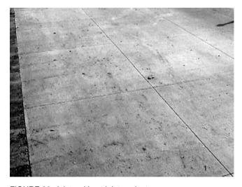
FIGURE 26 Joints without joint sealant.
