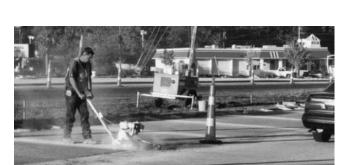
FIGURE 24 Sawcutting on a fast-tracked UTW.
