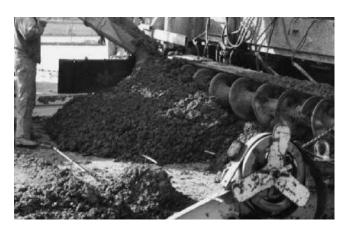
FIGURE 12 Use of a slipform paver.
