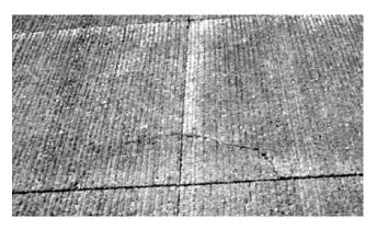
FIGURE 30 Typical corner crack on a UTW.
