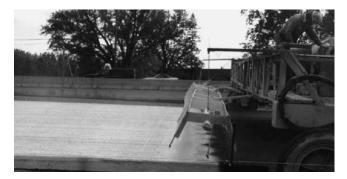
FIGURE 22 White-pigmented, liquid membrane curing compound.
