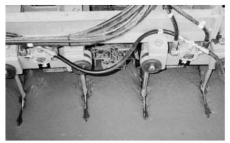
FIGURE 16 DBI submerging dowels.
