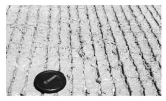
FIGURE 21 Tining comb texturization on freshly placed concrete.
