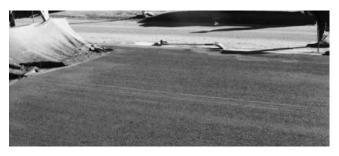
FIGURE 19 Application of texture with a burlap drag.
