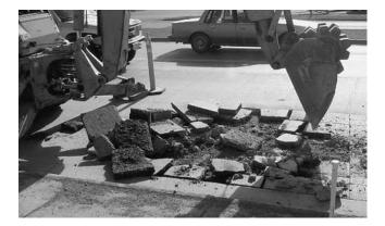
FIGURE 39 UTW repair step 2-Removing panels.
