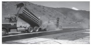
Colorado DOT rehabilitated runways at Glenwood Springs Municipal Airport by laying rubber-modified asphalt incorporating 5,000 scrap tires, which reduces community tire disposal problems and may save money on airport pavement rehabilitation.
