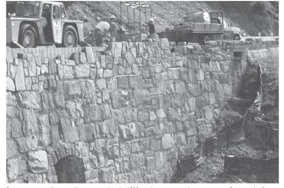
Stone masonry walls, originally constructed in the 1920s, undergo repair and maintenance at Going-to-the-Sun Road, Glacier National Park, Montana.
