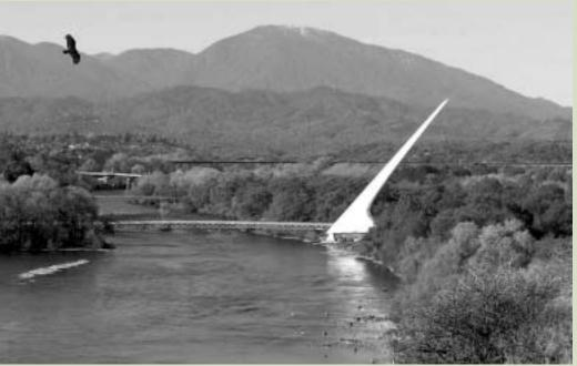
and transported by truck to Redding. The parts, supported by cables stretched from the pylon, were welded together above the water. For further information visit www.turtlebay.org/bridge/index.html.
