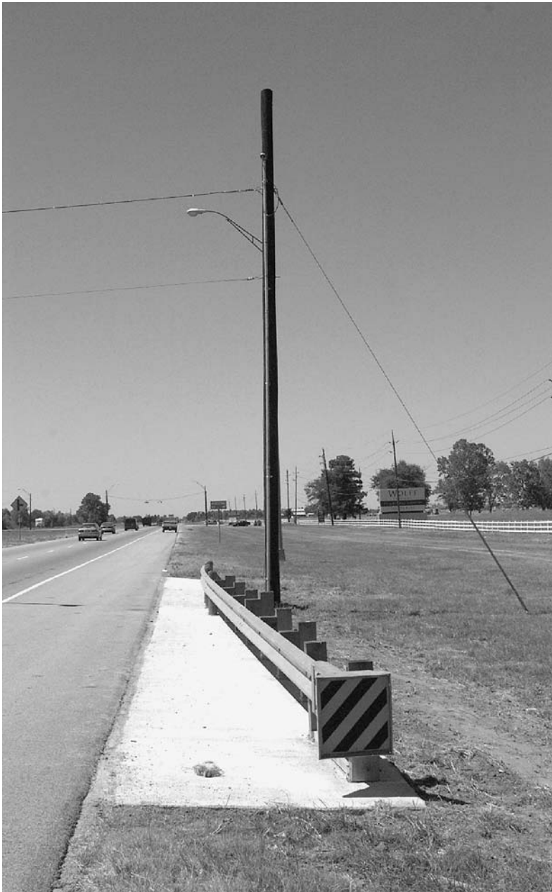
FIGURE 3 Extruder terminal and guardrail (guardrail installation on pole).
