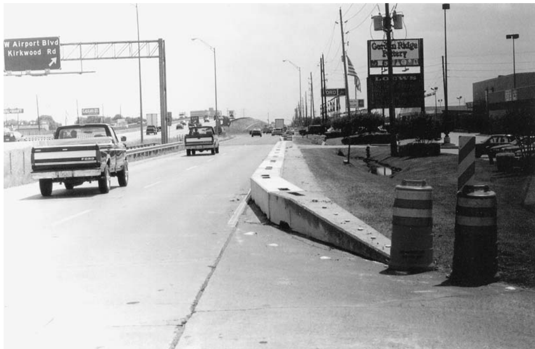
FIGURE 2 LPB, construction zone.
