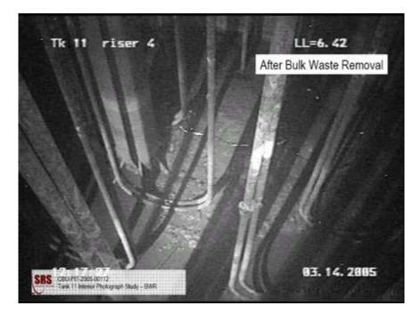
FIGURE 5 A Type I tank (Tank 11) after undergoing bulk waste removal in March 2005. SOURCE: Caldwell (2005b).
