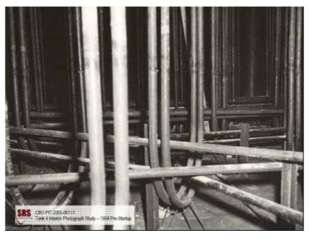
FIGURE S-1 Photograph of the interior of a Type I tank (Tank 4) prior to receipt of wastes. SOURCE: Caldwell (2005a).
