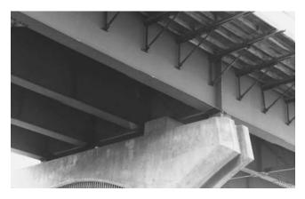
FIGURE 2 Deck cantilever brackets (DeLong's Inc.).
