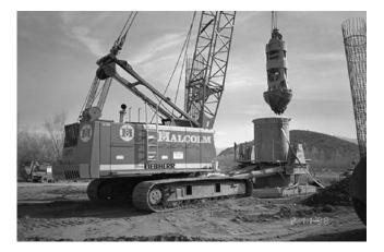
FIGURE 49 Casing oscillator and hammergrab tool.
