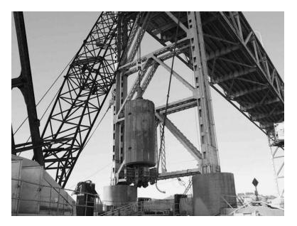
FIGURE 57 Shrouded bottom hole assembly lifted for placement through the top unit (Byles 2004).
