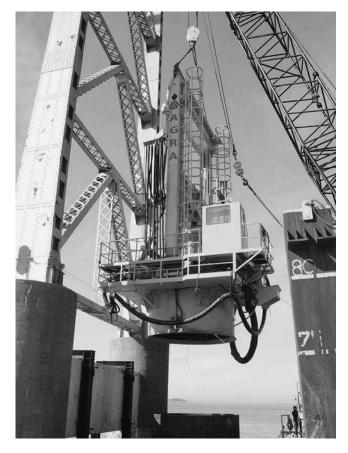
FIGURE 56 Toredo T40-4 pile top unit being placed over casing for reverse circulation drilling, Richmond–San Rafael Bridge (California) (Byles 2004).
