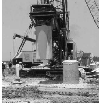
FIGURE 48 Intact rock core removed using crane-mounted rotary drill and core barrel.
