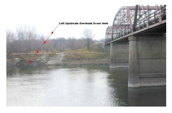
Figure 6. Looking at left upstream overbank scour hole (inside what appears to have been a much larger scour hole) from right bank along the upstream bridge face of S.R. 25 over the Minnesota River during low-flow.
