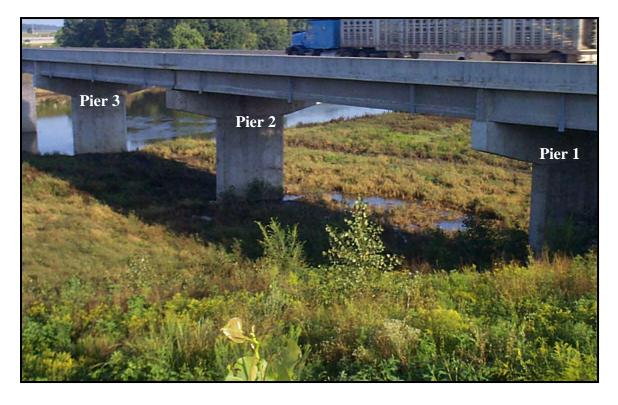
Figure 12. Looking upstream at left overbank and areas of clear-water scour from downstream US 218 bridge over Cedar River during low flow, 8/10/99.
