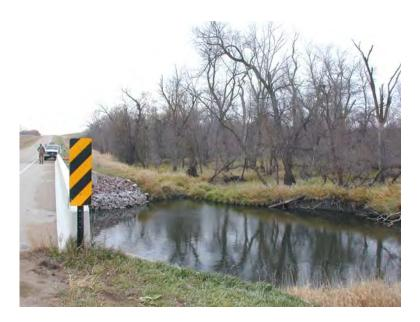
Figure 6. Looking at scoured area on right upstream bank of County Route 22, during low flow.
