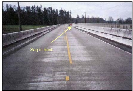
Figure 10. Looking west toward sag in bridge deck due to failure of pier #9 during the February 1996 flood.
