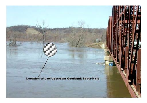
**Figure 5.** Looking at flow contraction from left floodplain and location of upstream left overbank scour hole from right upstream abutment of S.R. 25 bridge during April, 2001 flood.
