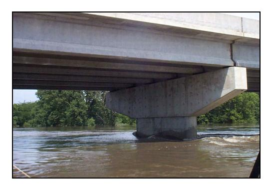
**Figure 6.** Looking upstream at wake around Pier 5 of upstream US 218 bridge over the Cedar River, 7/23/1999.
