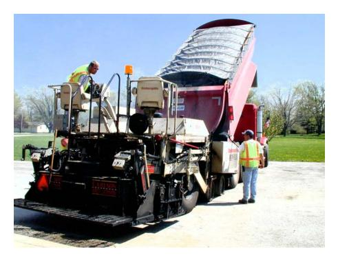
Figure D.2 Loading the paver
