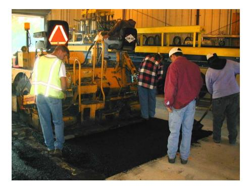
Figure D.4 Test section paving
