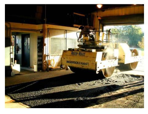
Figure D.5 Mixture compaction
