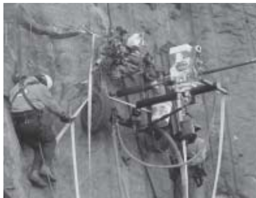
Overcoring to exhume rock reinforcement.
