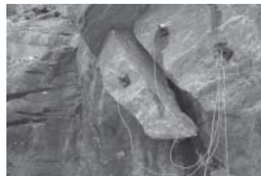
Rock bolts wired for nondestructive testing.
