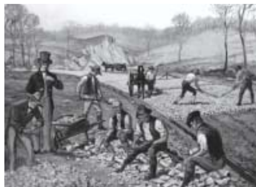
The National Road was the second U.S. road to use the McAdam principle of compacting broken pieces of rock that weighed less than 6 ounces and were smaller than a 2-inch ring; the process took 5 years to pave 73 miles by 1830. (Detail from painting by Carl Rakeman, courtesy of FHWA.)
