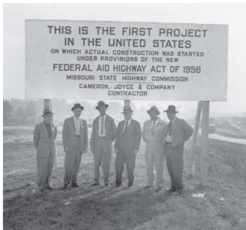
On August 2, 1956, Missouri became the first state to award a contract with the new Interstate construction funding. Of three contracts signed that day, the Missouri State Highway Commission first authorized a contract for work on U.S. Route 66—now Interstate 44—in Laclede County; the other contracts were for work on U.S. 40—now I-70, the Mark Twain Expressway—in St. Louis and for another section of the highway in St. Charles County. Work started August 13.
