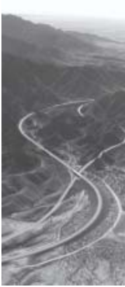
Telegraph Pass, Interstate 8, near Yuma, Arizona.
