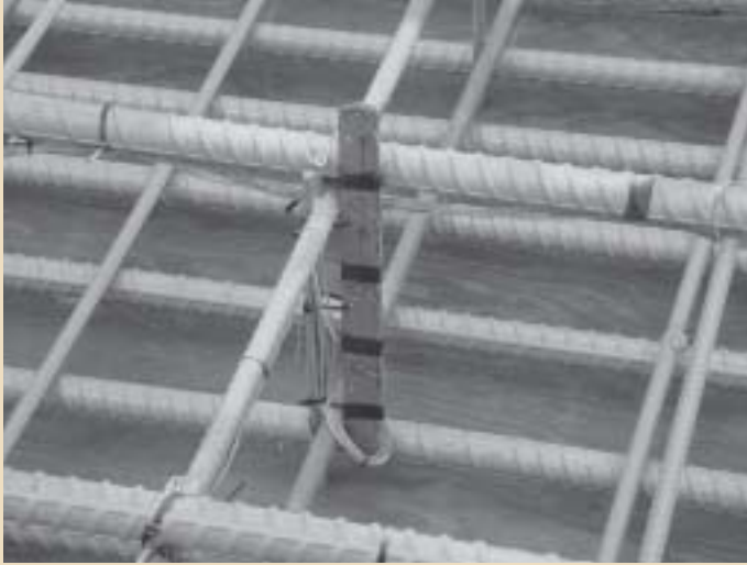
I-button electronic device installed on an Interstate 70 bridge to record pavement temperatures; the data assist in modifying concrete curing specifications to increase durability.
