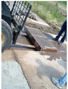
Figure 7. Removal of the Asphalt Test Section at Mn/DOT's Mn/ROAD Facility
