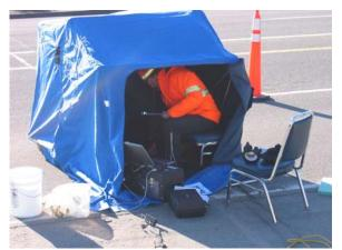
Figure 15. Ice Fishing Shelter Tent Installed over Pavement Sensor
