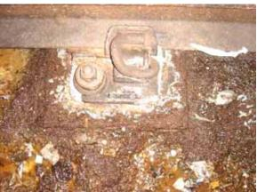
TTC-Toronto tracks showing deposited salts and resulting corrosion.
