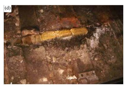
PATH Transit System showing (a, b) rail corrosion, (c) ice spikes from sealant used to prevent water leaks in the tunnel, and (d) salts deposited along the tracks. Note: The site visit was conducted during January 2006 and due to the weather conditions in New York and New Jersey, the water leaks froze forming the ice spikes shown in photo (c).
