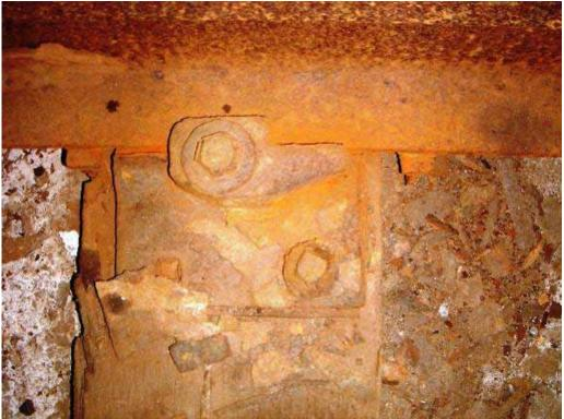
Rail donated by Amtrak (Baltimore) and a location on the tracks showing severe corrosion.
