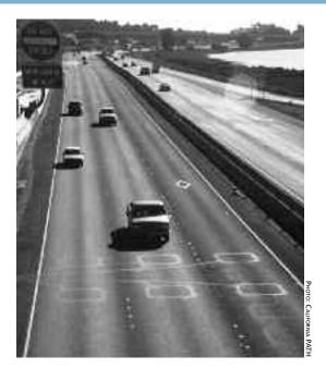
Loop detectors in highway pavement can generate data on traffic conditions and travel time.
