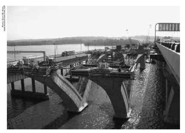
Construction of the new Woodrow Wilson Bridge on I-95 and I-495 across the Potomac River near Washington, D.C., proceeded as traffic continued on the old bridge (*left*) and on the completed span (*right*).
