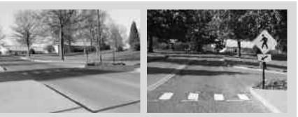
A road safety audit identified a crosswalk (left) not visible to approaching motorists. A sign was installed to indicate the location of the crosswalk clearly (right) and to enhance pedestrian safety.
