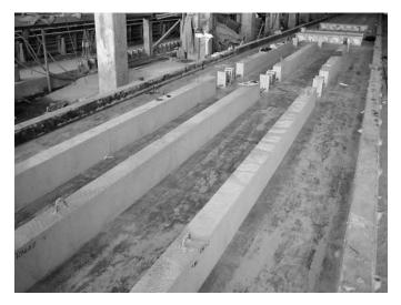
Figure 3.17. Fabrication of rectangular beams.
