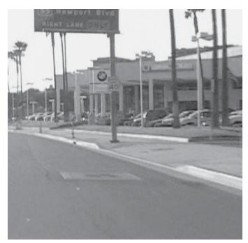
Photo by Karen Dixon. Figure 20. Lack of positive guidance at a driveway.
