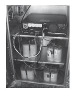
Installation of UPS in a separate, attached cabinet; the UPS unit is on the top shelf, and the batteries are on the middle and bottom shelves.
