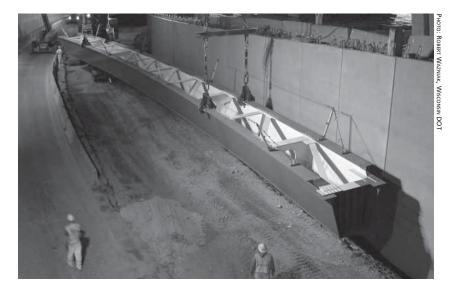
Contractor lifts a tub girder into place for the connector ramp between I-94 Westbound and I-43 Northbound, one of several innovative construction methods employed to ensure rapid completion of the interchange project.
