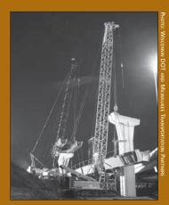
COVER: A curved steel box girder is placed on one of the system ramps at night during reconstruction of the Marquette Interchange in Milwaukee; communication and collaboration with stakeholders was a key to the successful completion of the project.
