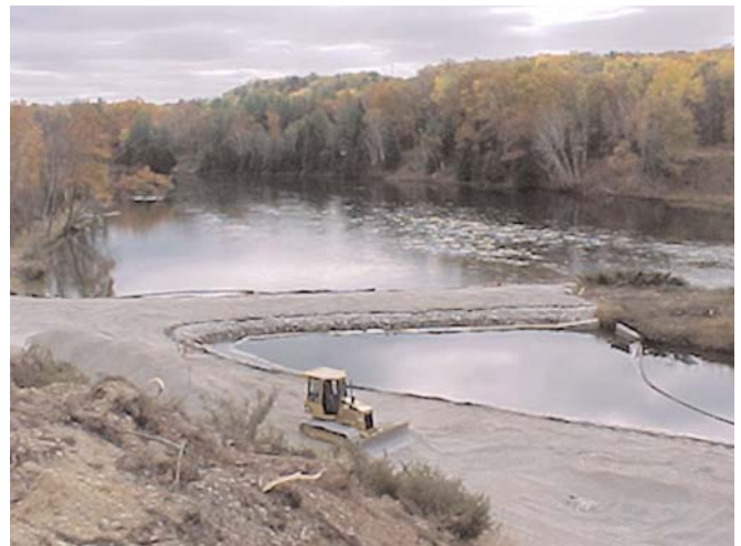
Figure 4 Temporary causeway fill with filter fabric, sheet piling, and concrete barrier used in Michigan.
