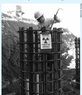
Technician with Caltrans Foundation Testing Branch inserts a gamma-gamma logging probe over rebar cage for a drilled shaft.
