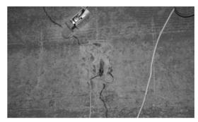
Cracked RCDG bridges were instrumented and monitored.
