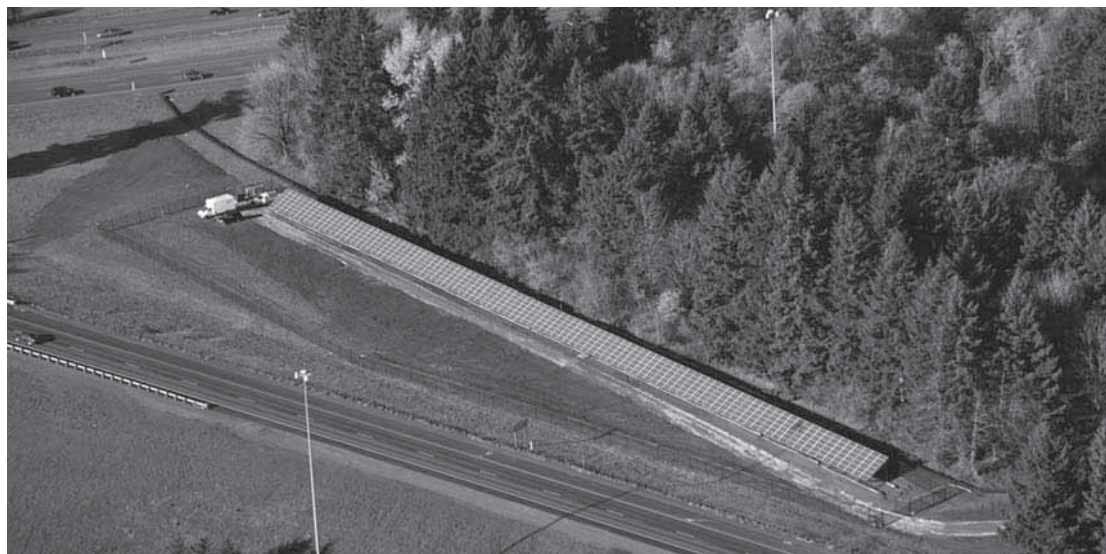
A ground-mounted array of 564 solar panels at the intersection of Interstates 5 and 205, near Tualatin, Oregon, generates 28 percent of the power required to light the interchange at night and reduces pollution.
