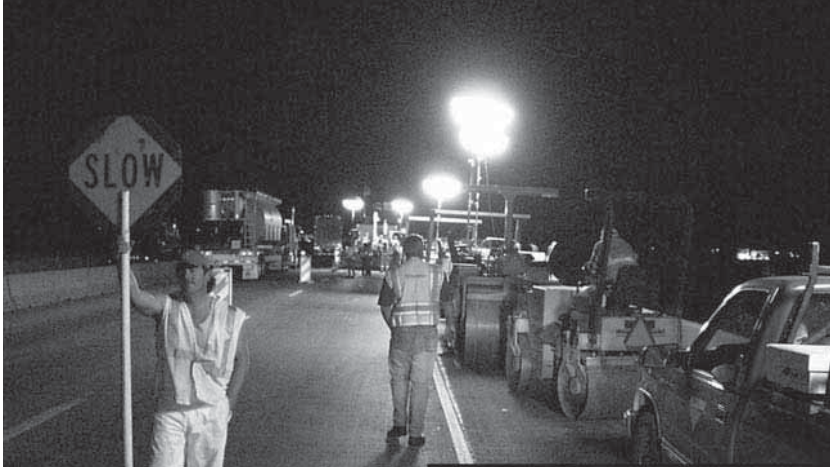
Balloon lighting in use on paving equipment.
