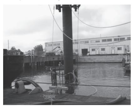
Caltrans also conducted tests on sound reduction methods that had been developed to protect marine mammals. The underwater sounds during this demonstration, however, fatally injured fish, which were observed floating on the surface and exposed to predation by seagulls. Because the sound reduction methods were not protecting the fish adequately, state and federal agencies raised concerns about the endangered fish species in the area.
