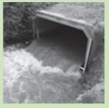
A concrete box culvert in a medium- to high-gradient mountain stream. The culvert width is less than the width of the stream channel; therefore, during high flows, as shown in the photo, the constriction creates a velocity barrier to the upstream passage of most fish species. Because the water velocities also create scouring downstream, the culvert includes an outlet drop, which fish must negotiate in addition to the water velocities within the structure.
