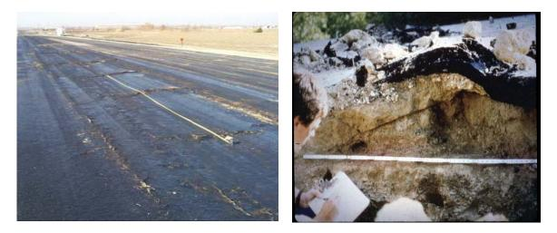
Figure 5. (a) Evidence of failures due to the accumulation of lateral strain due to sulfate-induced expansion (43) and (b) accumulation of considerable lateral strain resulting in shear failure in lime-treated high sulfate soil layer (Photograph courtesy of Dr. Thomas Petry).
